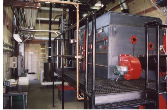
The wood waste boiler supplies heat for the kilns, and produces enough excess steam for a turbine generator to provide 150 kW of electricity for the facility.
